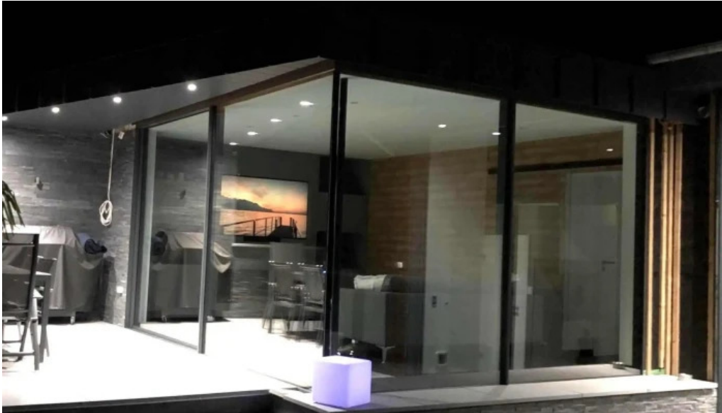
Keller minimal windows ulflingen
