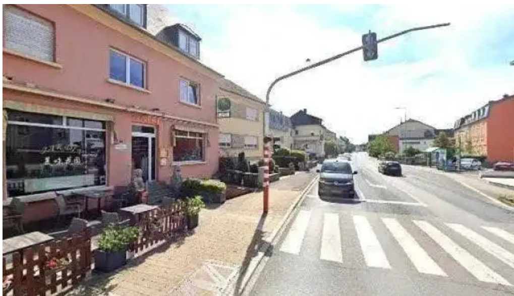
Crlux construction locatione
