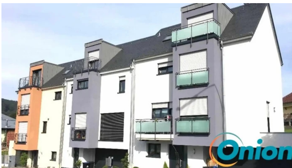
Siebenaller constructions remisene
