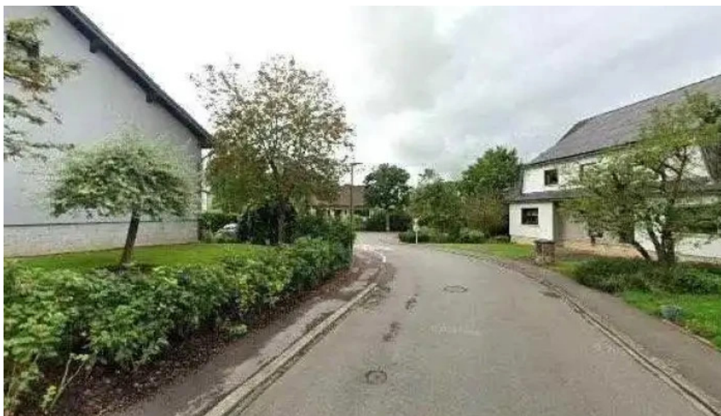
Bm constructions street view 360deg fotos
