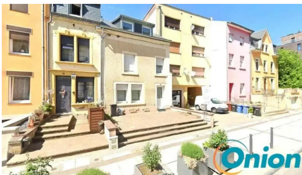
Artconstruction sarl Differdange
