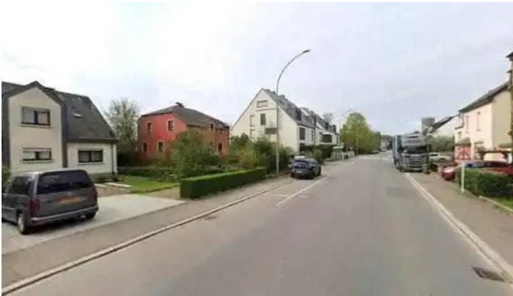
Marsant constructions sarl street view 360deg fotos
