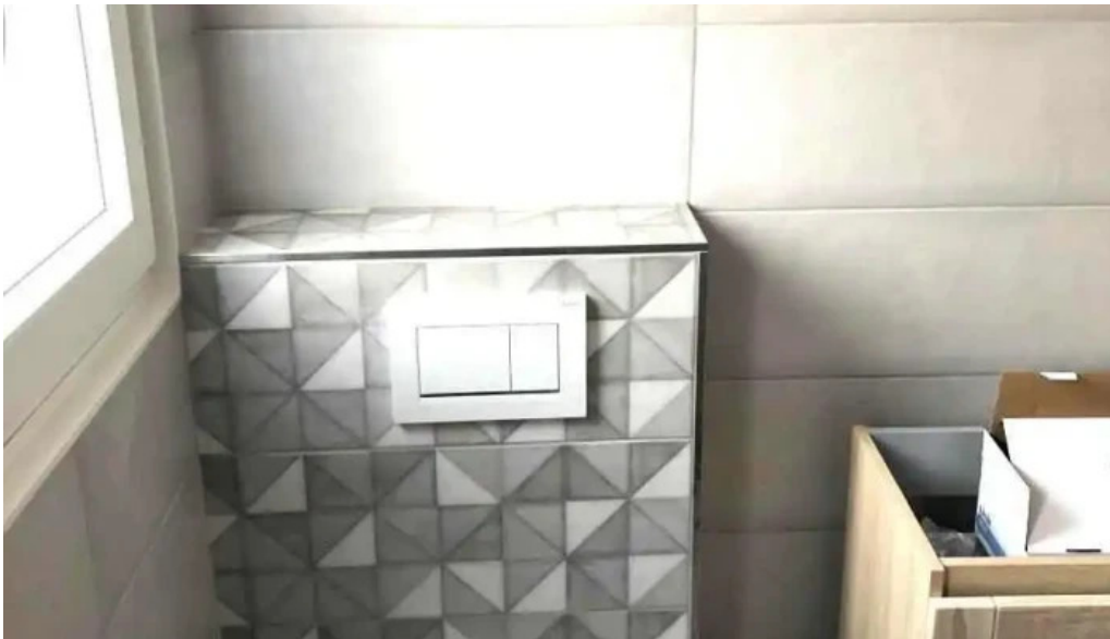
Kintziger concept construction innenansichten
