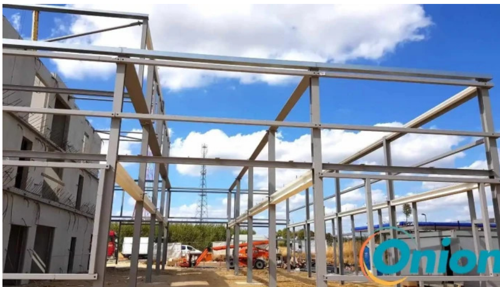
Cement construction steinsel
