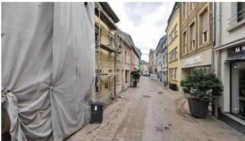
Abattage theis grosges sarl street view 360deg fotos
