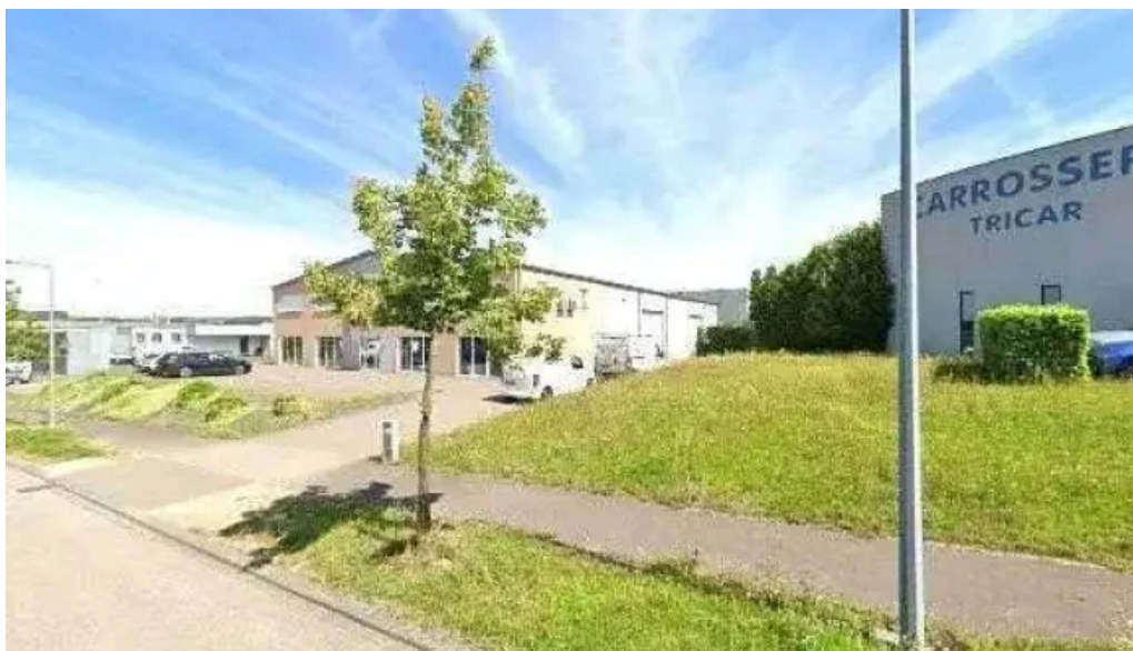
Hoen sarl construction facades street view 360deg fotos
