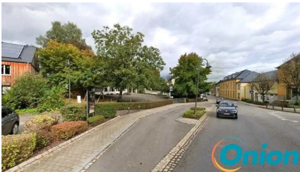
Electricite electro watt s a beckerich
