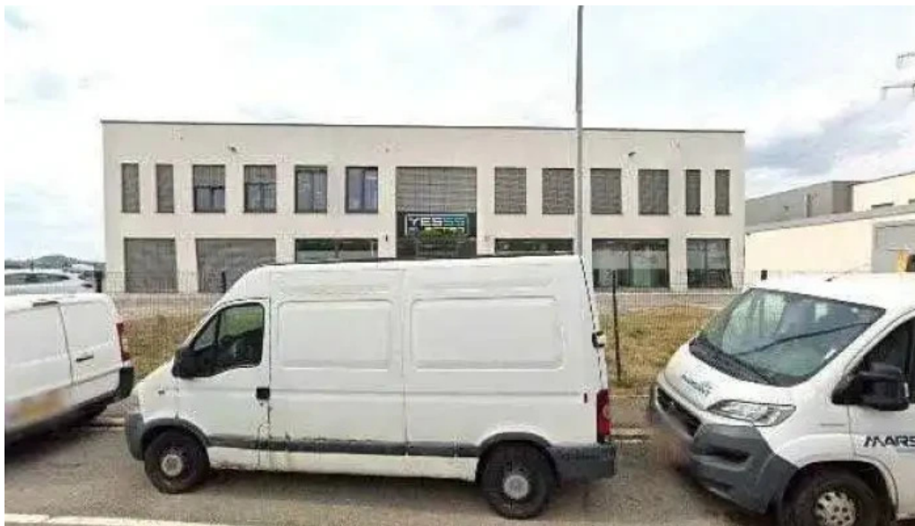
Yesss electro street view 360deg fotos
