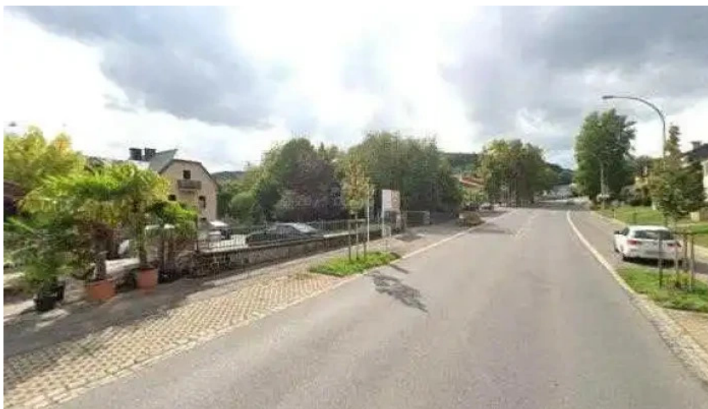
Nettoyage olaf stein sarl street view 360deg fotos
