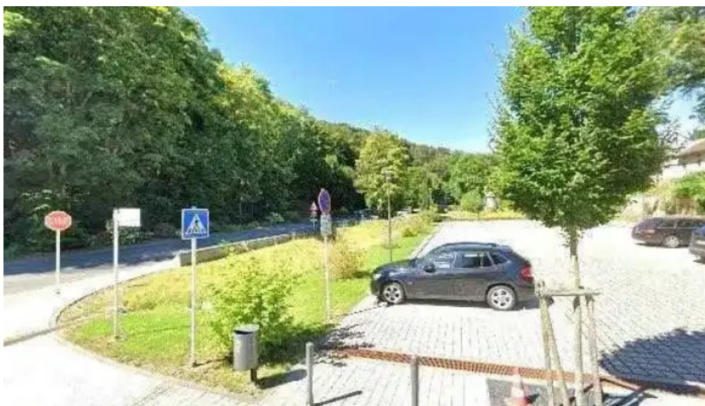
Swio ladestation telephone
