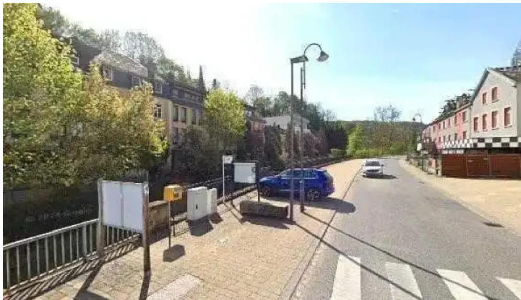
Totalenergies charging station locatione
