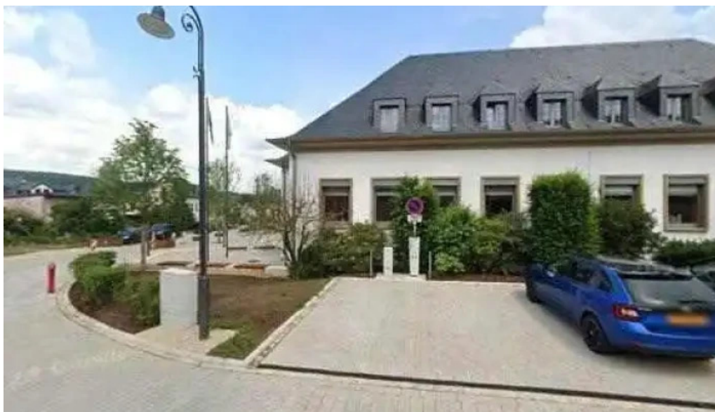
Chargy charging station bewaertunge
