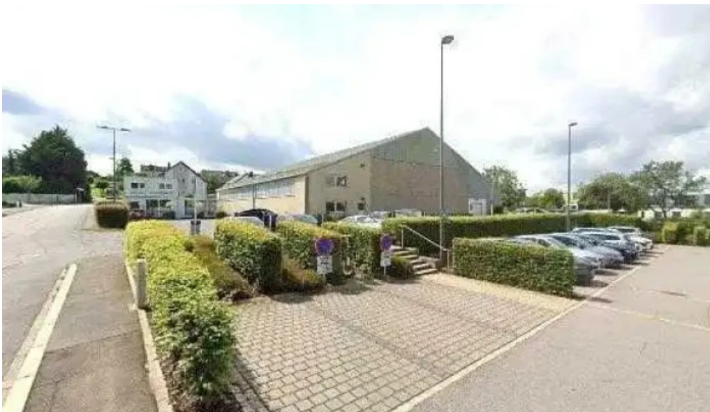
Chargy charging station geigende
