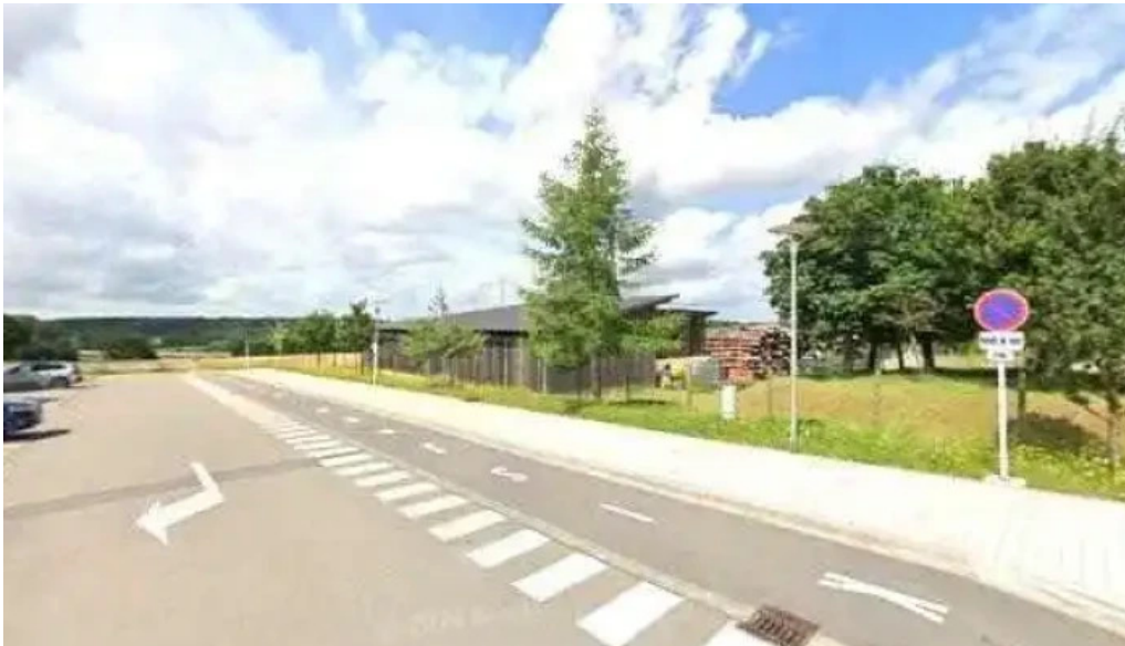
Chargy charging station remisene
