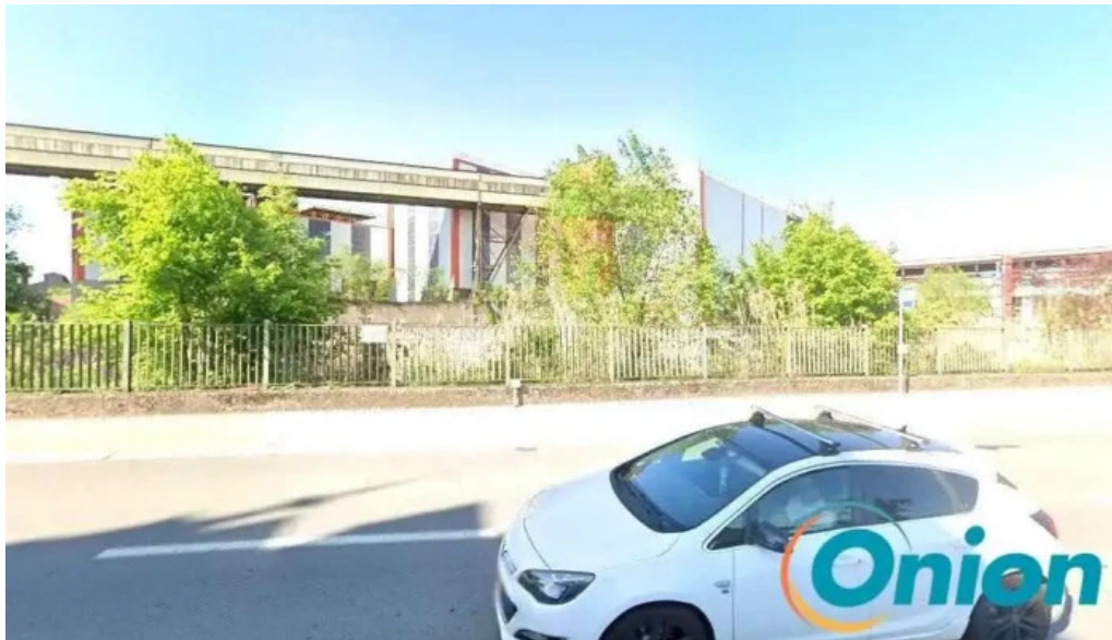
Evbox charging station differdange
