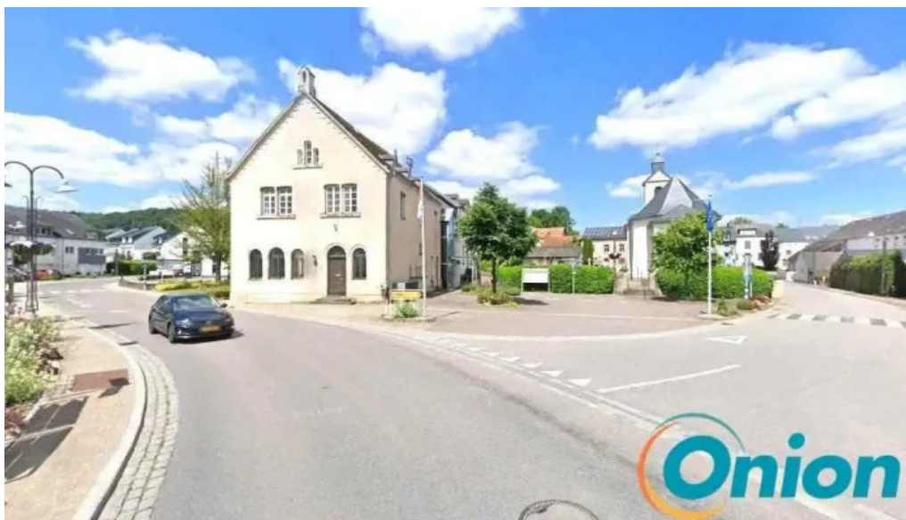
Chargy charging station flaxweiler
