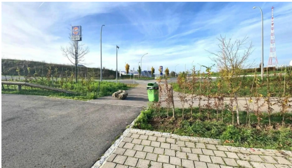
Chargy charging station street view 360deg fotos
