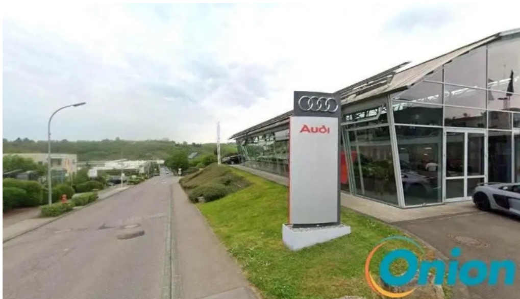
Losch import sarl charging station junglinster
