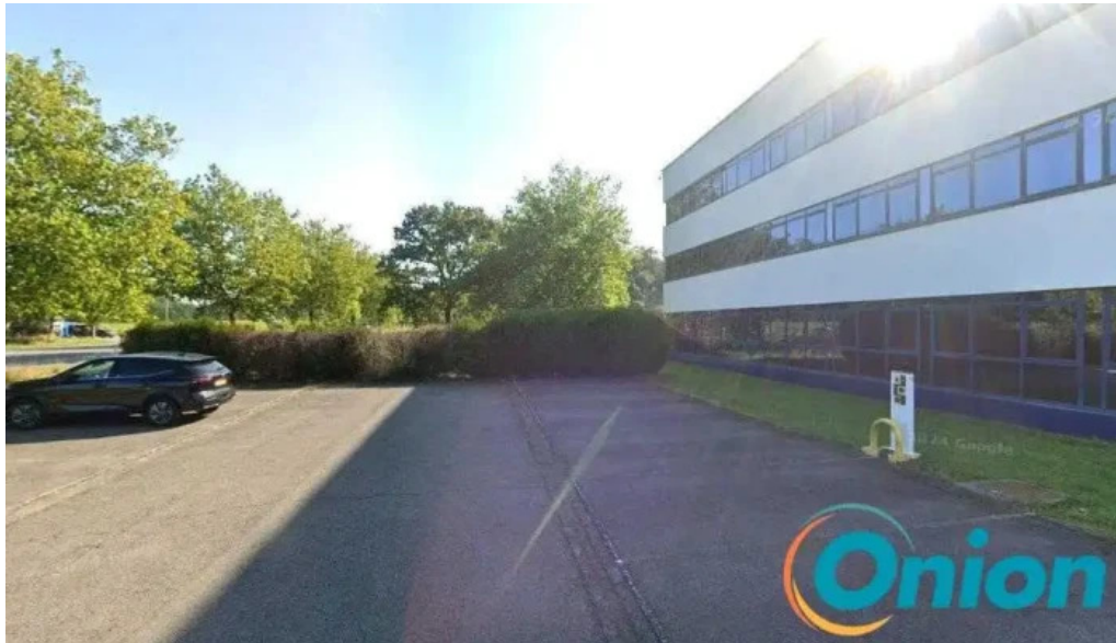
Chargy charging station kaerjeng
