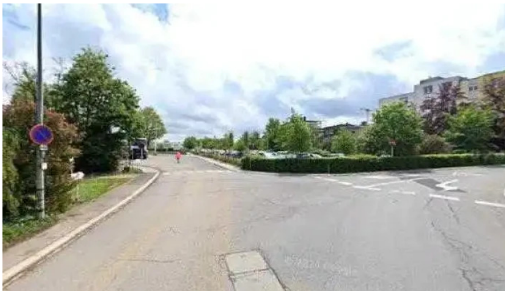
Chargy charging station promotioun
