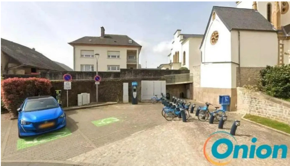
Chargy charging station mamer
