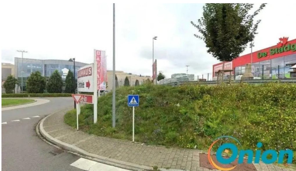
Electric vehicle charging station mamer
