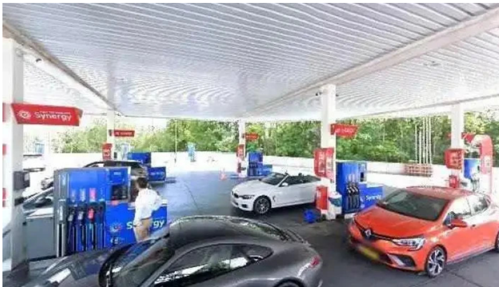
Bestcharge ladestation street view 360deg fotos
