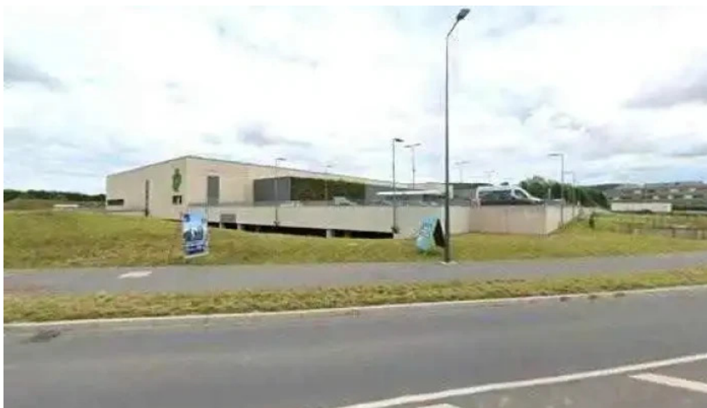
Chargy charging station geigende
