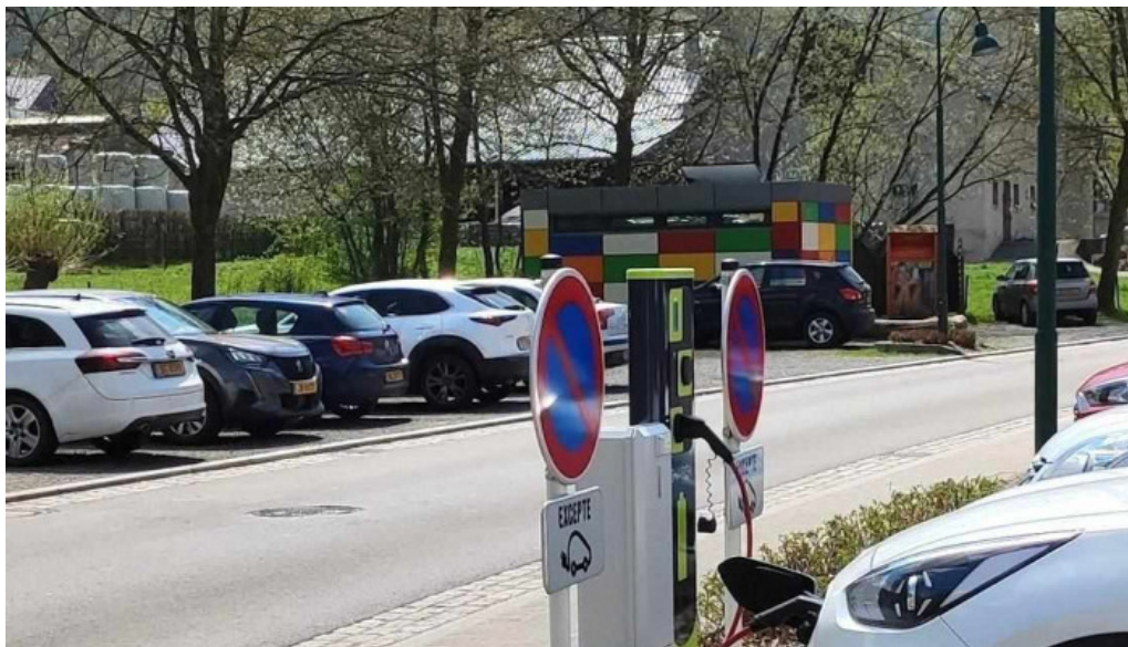
Charge charging station bewaertungene
