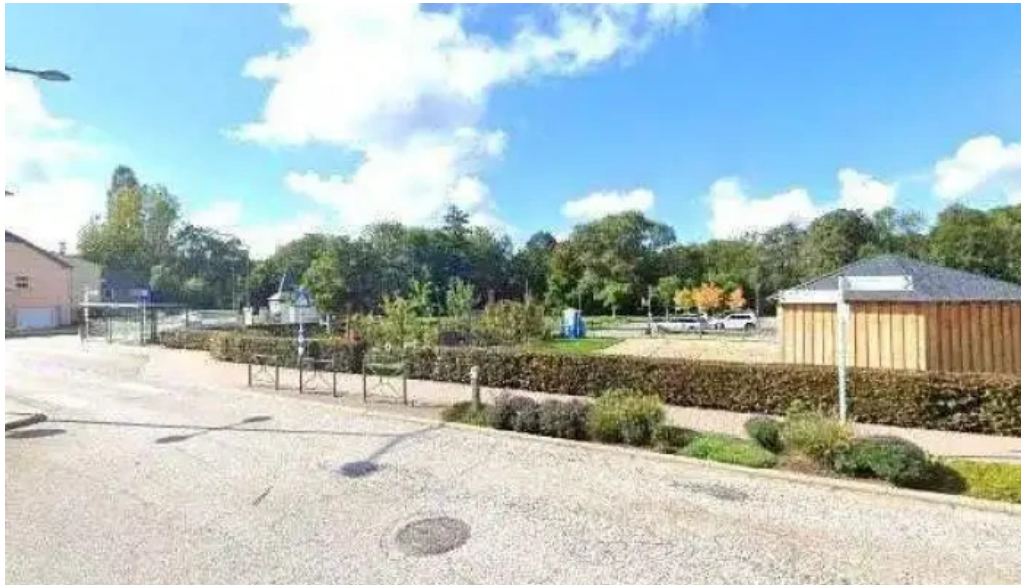
Innogy charging station wei do ukommene
