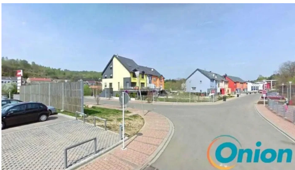
Totalenergies charging station rumelingen
