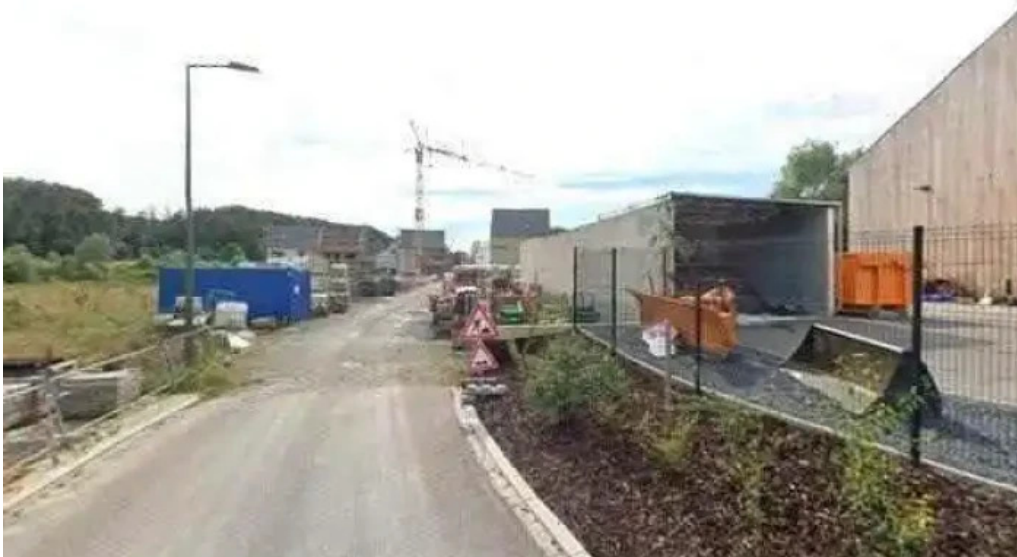
Chargy charging station street view 360deg fotos
