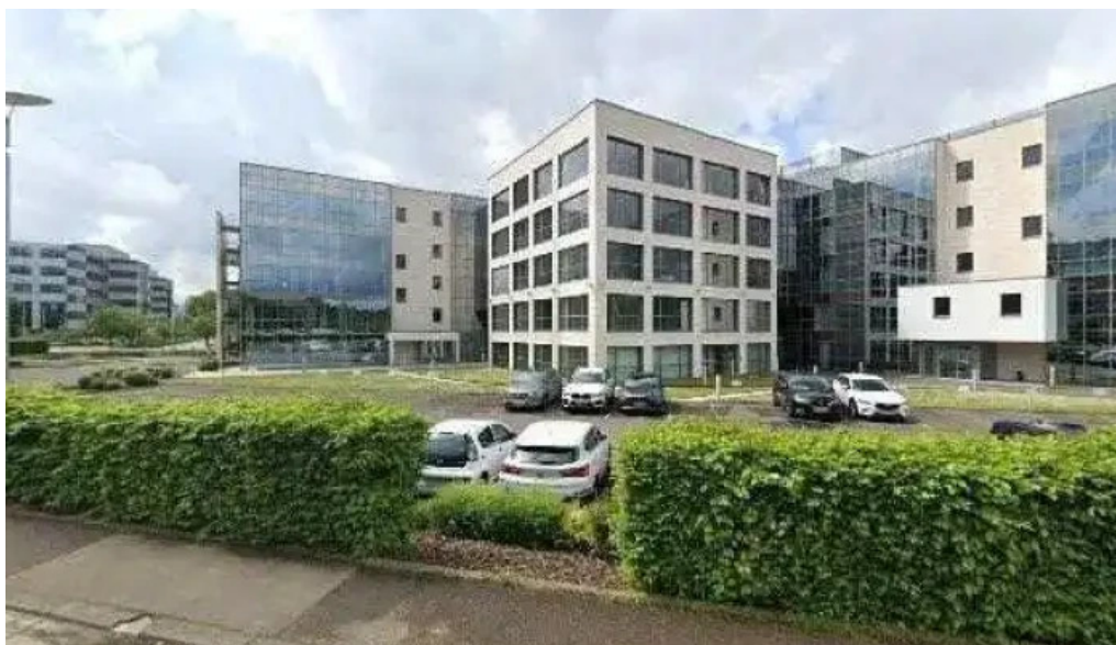
Chargy charging station remisene
