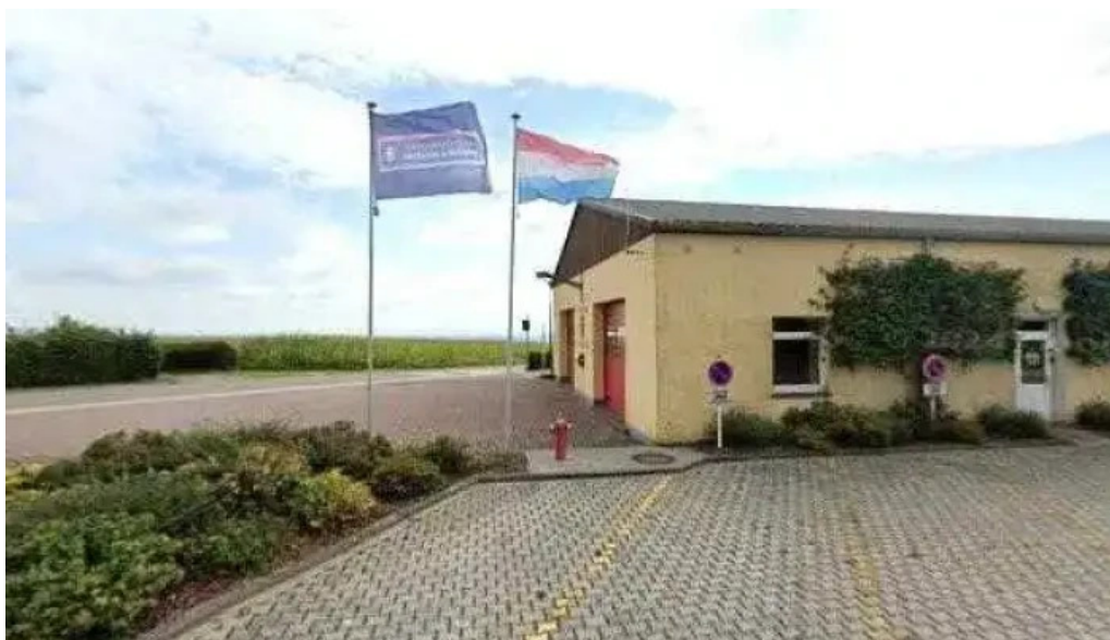
Chargy charging station stonnenplange
