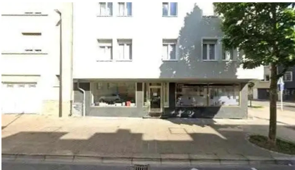
A2 peinture facade street view 360deg fotos
