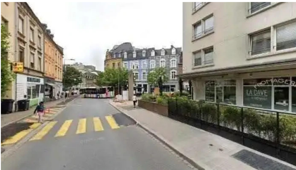
Upside projects street view 360deg fotos
