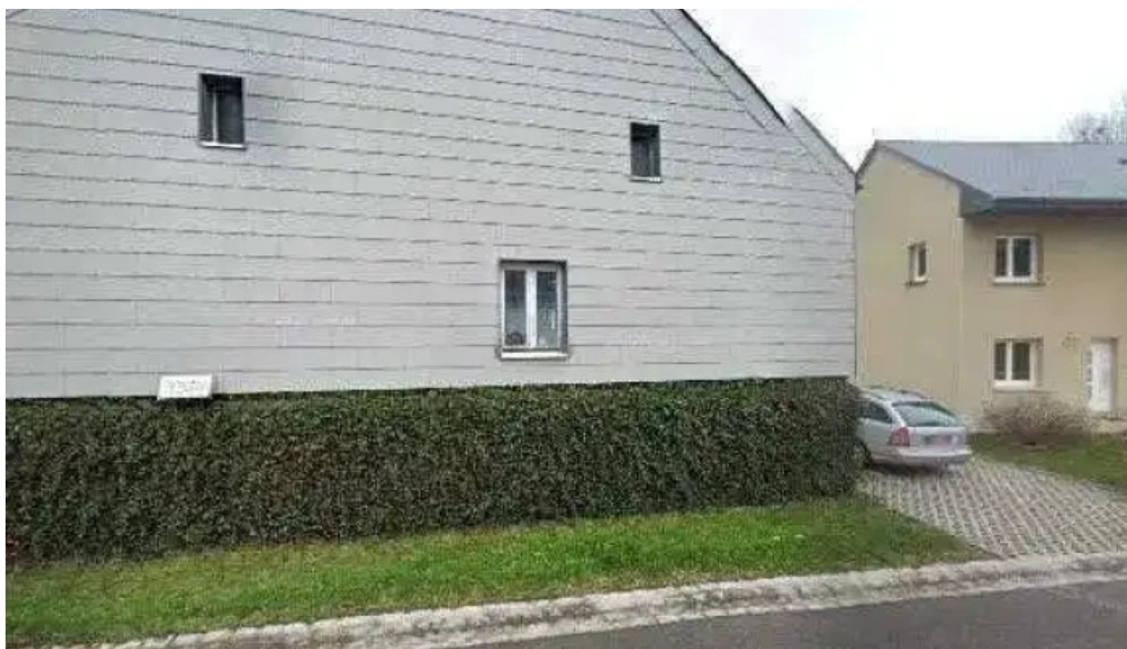
Advensys constructions sarl street view 360deg fotos
