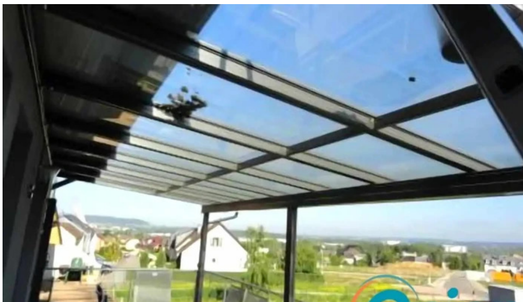
Via nettoyage differdange
