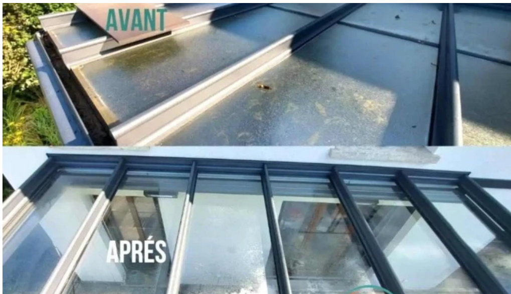
Gni services sarl innenansichten
