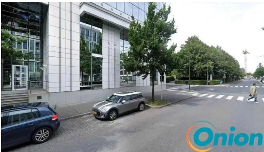
Cable wireless luxembourg sa luxembourg
