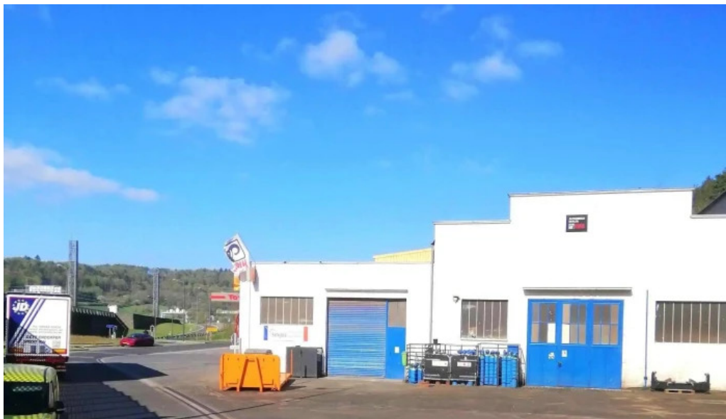
Totalenergies lorentzweiler location
